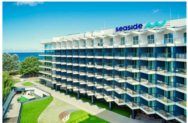
Building: Seaside Park Hotel Country: Poland City: Kolobrzeg
