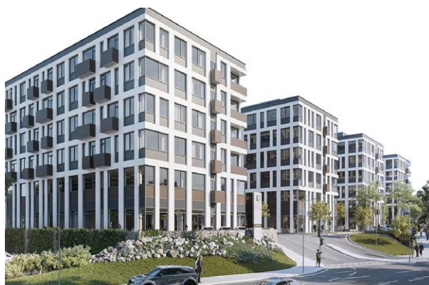
Building: Omnia 2000 Country: Czech Republic City: Bratislava Units: 25 (VENTUS VVS, VENTUS Compact)
