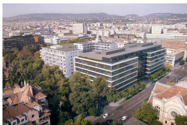
Building: Green Court office Country: Hungary City: Budapest Units: 12 (VENTUS VVS)
