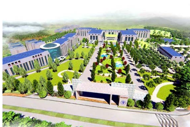
Building: AIIMS Bilaspur, Country: India City: Himachal Pradesh, Units: 130 ( VENTUS VVS)
