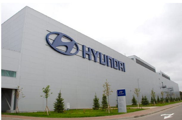
Building: Hyundai motor manufacturing Country: Russia City: Saint Petersburg
