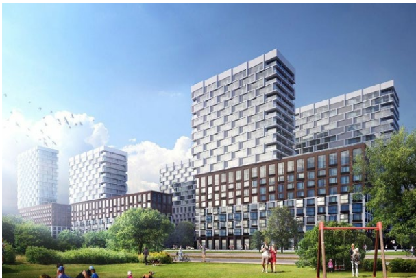
Building: Sobyitie residence complex Country: Russia City: Moscow
