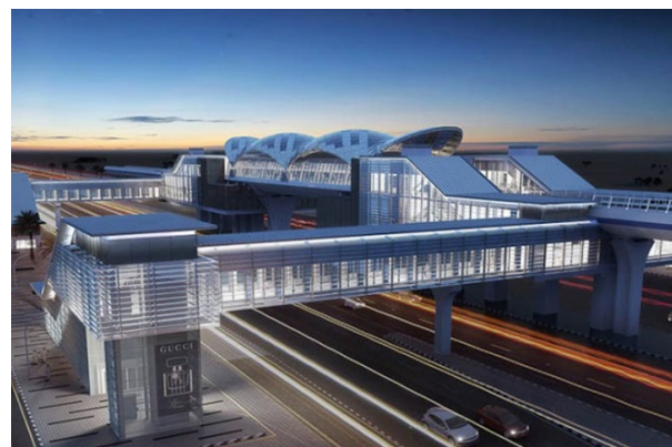
Building: Riad Metro-Package 3 (Line 4,5,6) Country: KSA City: Riyadh
