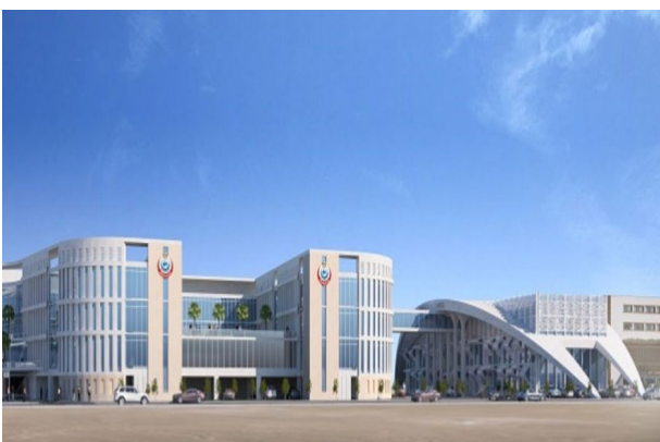
Building: Suez Complex Country: Egypt City: Suez
